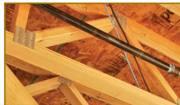
Thermal Bypass Inspection
